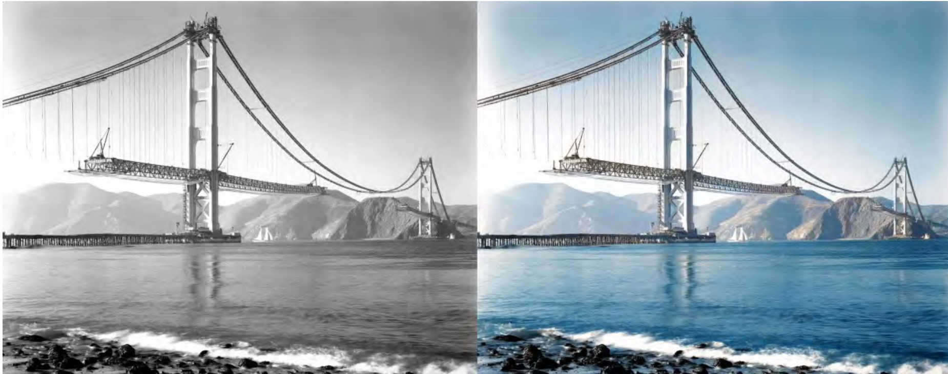
A deoldified Golden Gate Bridge under construction.
