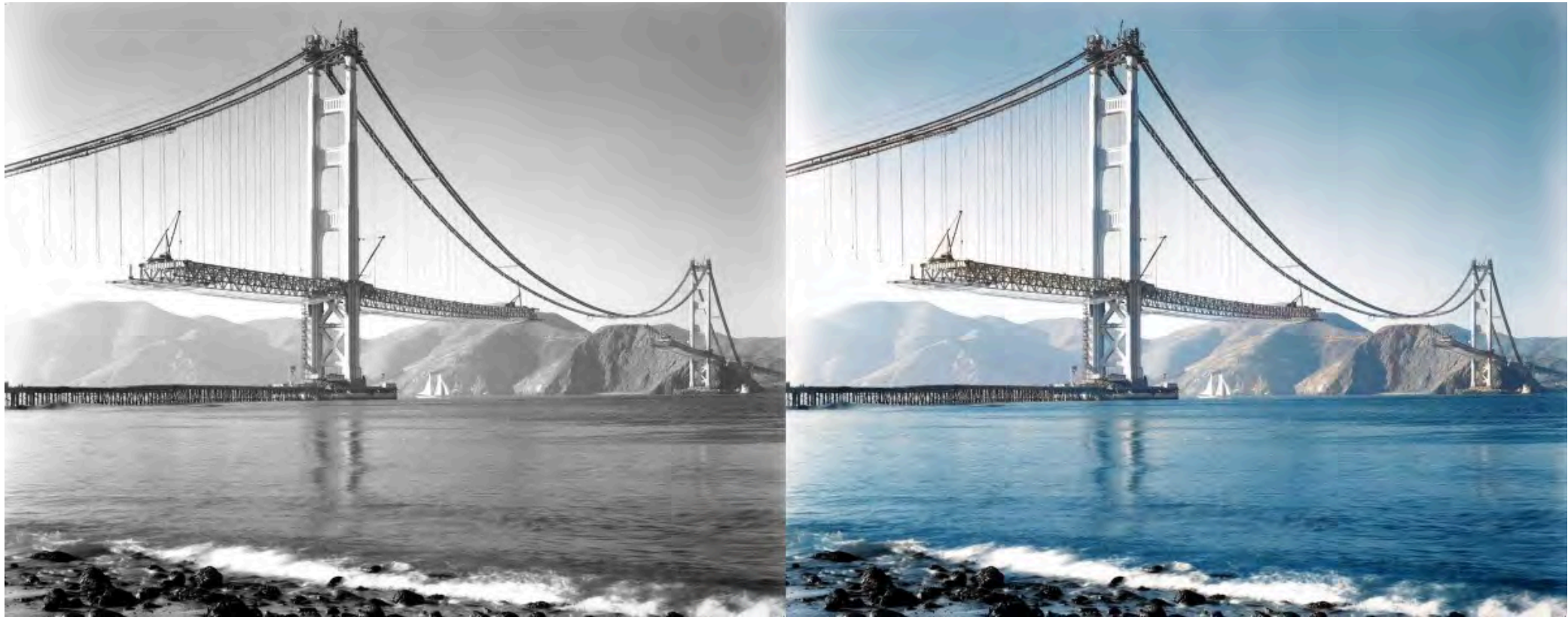
A deoldified Golden Gate Bridge under construction.
